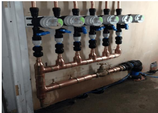
[Example: Individual meters downstream of a boosted storage cistern]
