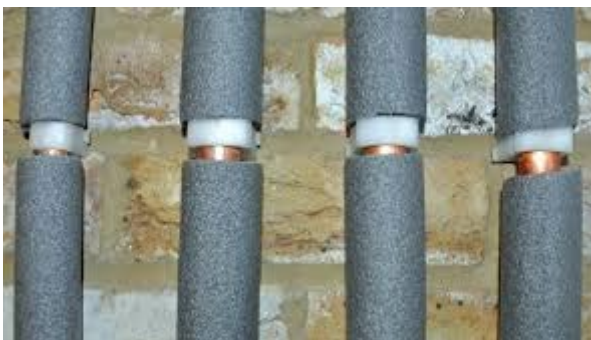
[Expanded Rubber Nitrile Insulation such as Armaflex O - Recommended within a duct at the point of entry. Minimum 19mm wall thickness but thicker required for a shallow point of entry]
