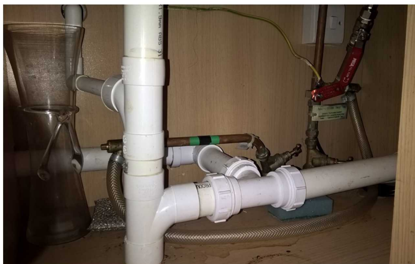
Figure 1 – Cross connection between rainwater and wholesome supply
